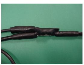
9) Apply one layer of butyl rubber mastic, overlapping the coax jacket by at least 1" on each end of the exposed outer conductor. Overlap each wind by one half of the width of the mastic. Cut any remaining mastic and dispose of it properly.
