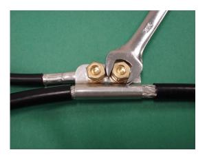
6) Cut four 2" pieces of butyl rubber mastic. Wrap a piece both above and below the ground clip as shown in the picture. Fold one of the 2" pieces of butyl rubber in half and place over the riveted ground lug and brass hardware to act as a filler. Wrap the final 2" piece of butyl rubber around the cable as shown.
